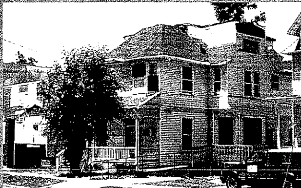
Originally built in the 1880s, this house showed the ravages of time. The time removed from the 1940s single-story, repaired wood siding and removal of metal siding restored the exterior of the house and helped it to look like the original. The original
