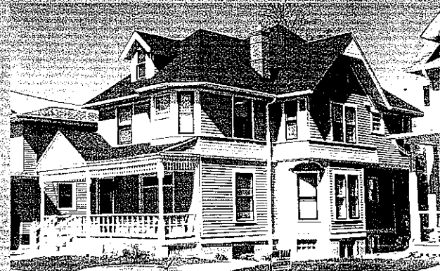
Originally built in the 1880s, this house showed the ravages of time. The time removed from the 1940s single-story, repaired wood siding and removal of metal siding restored the exterior of the house and helped it to look like the original. The original
